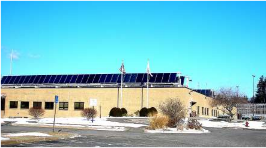
Hampshire County Jail and House of Corrections with PV Solar Cells on Roof
