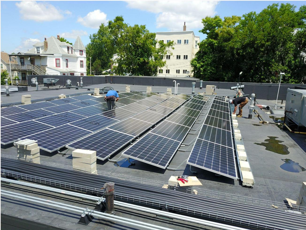
Example: 60 kW ballasted solar PV system installed at Commonwealth Kitchen, Dorchester, MA. The racking includes no penetrations and is weighed down on the roof to meet wind loading with cement blocks.
