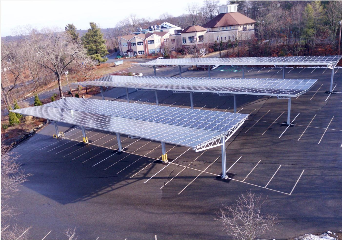
Example: 337 kW inverted truss solar PV canopy installed at Temple Emunah (Lexington, MA). This racking type covers parking spaces while leaving aisles open to maintain sunlight access for users.
