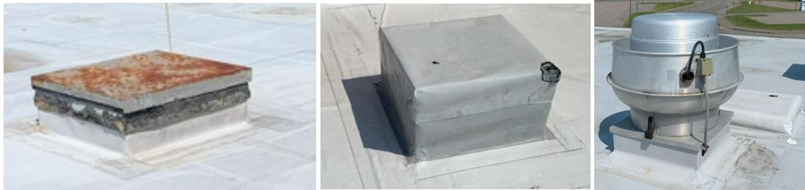
It should be noted that the white EPDM roofing membrane is in poor condition with many leaks and will require replacement soon.
