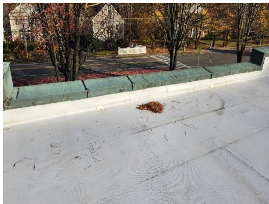
Typical view of EPDM Roofing
