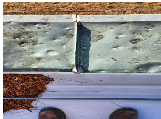
Typical view of Roof Parapet Coping Seam
