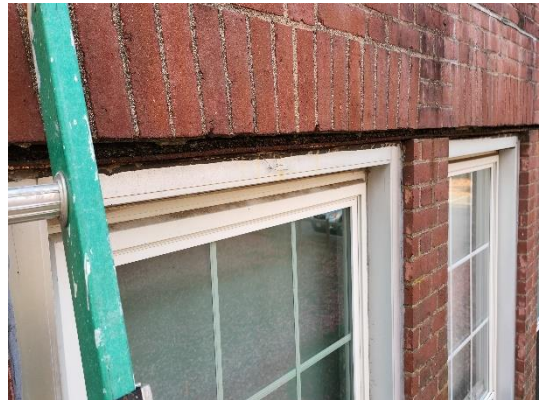
Typical East Wall Lintel Corrosion
