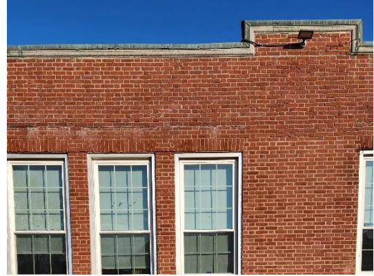
Typical West Wall Masonry Cracking
