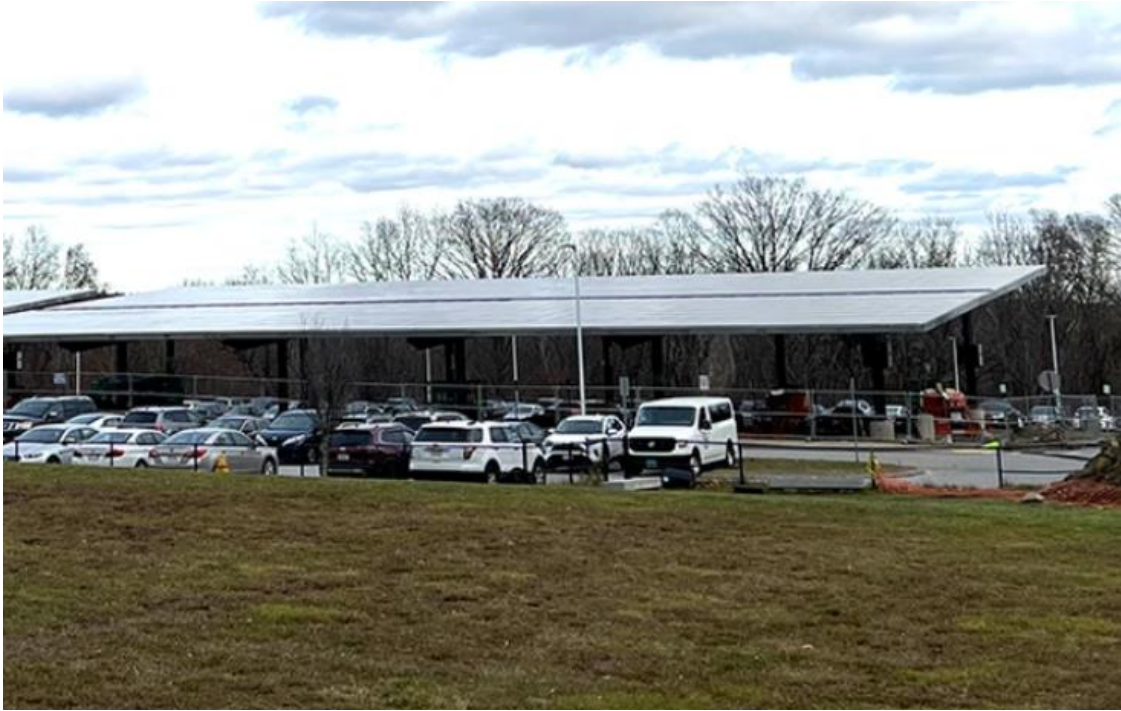
Canopies that cover the drive aisle
